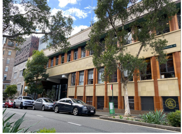
Figure 8: View of 80 Commonwealth Street 'Paramount Building'
