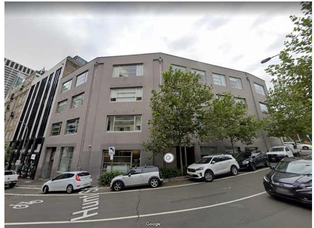
Figure 5: View of the site facing Hunt Street frontage (Source: Google Maps)
