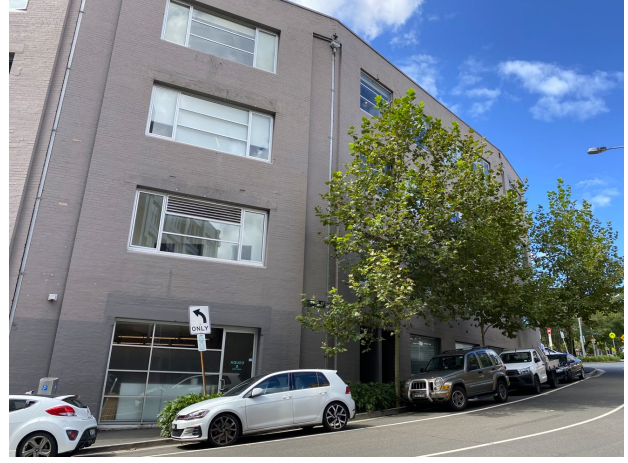
Figure 3: View of the site along Hunt Street frontage
